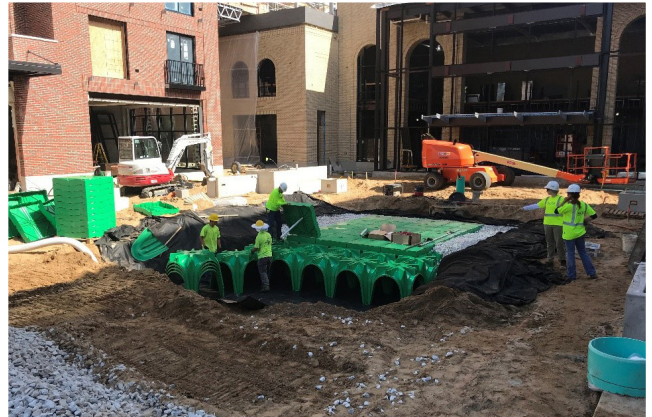
Triton Stormwater Solution’s new, revolutionary vault system is installed for the first time beneath this piazza.
